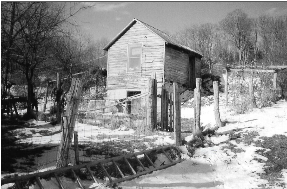
The Bryant smokehouse and ground cellar at their Fork Mountain farm
