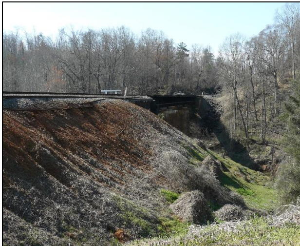
Train tracks over the Rockfish River
