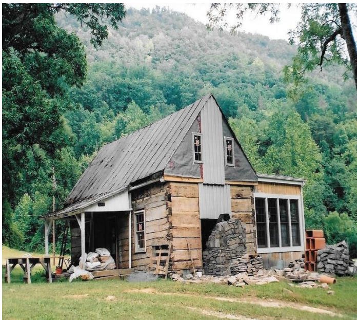
The Coffey chimney in the process of being built
