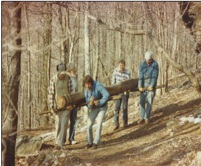
logs (for rafters, beams, and joists) were felled and hauled to the site, where they were worked and cut to shape; scaffolding was erected for work higher up.
