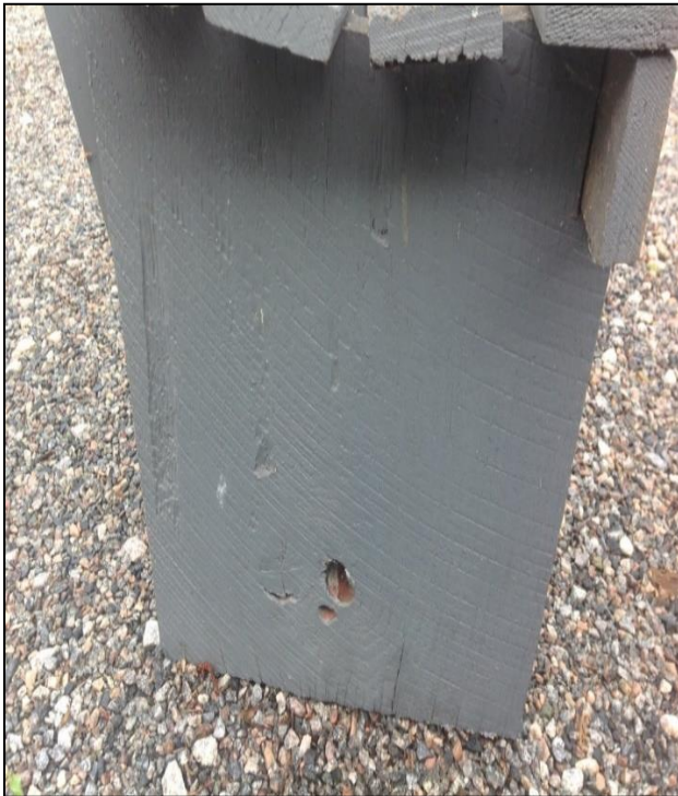
Circular saw mill marks on pew legs
