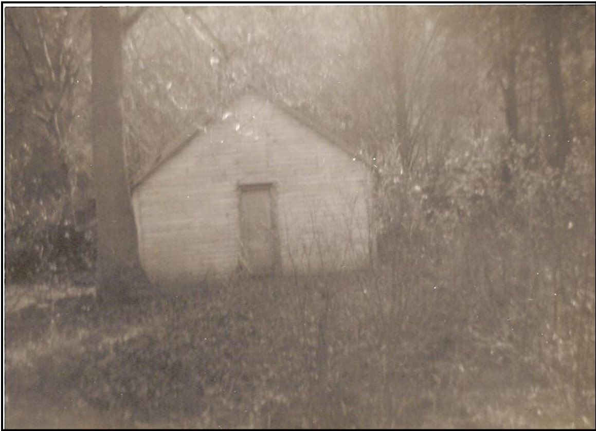
Church Building After Hurricane Camille – Lodged Against a Tree
