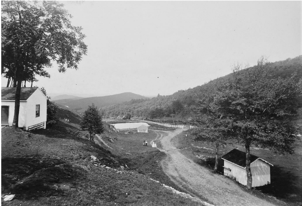
A view from the hotel porch looking north: pond in center of photo behind a small structure In 1969, when I-64 came through Afton Mountain, the pond was filled in (see next page)
