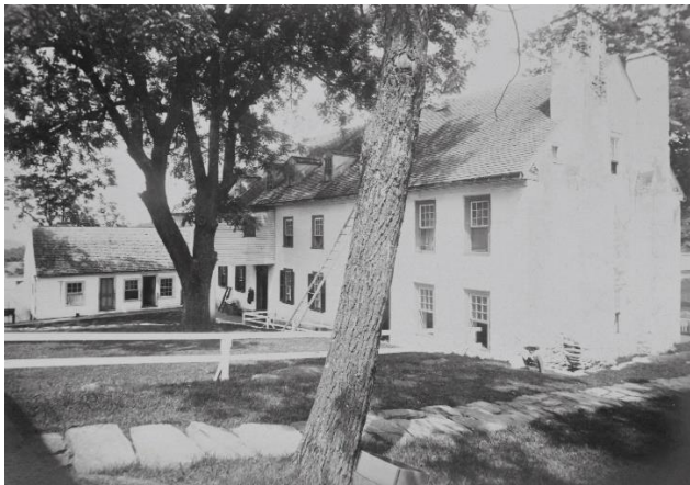
The rear of the Mountain Top Hotel
