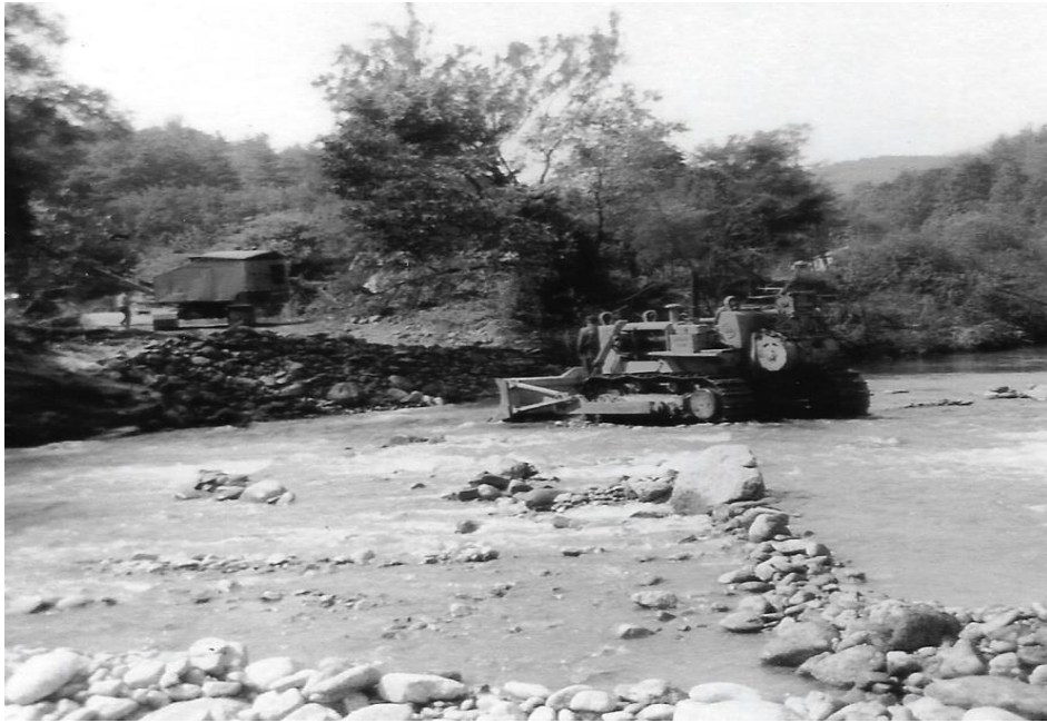
Large Equipment pushing rocks back into the Tye River after the flood
